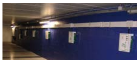
Image : Schneider Electric.
